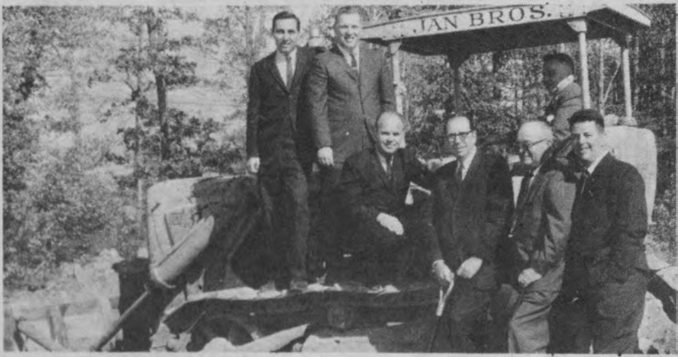
Madison Township; Ground breaking ceremonies for new plant for Frank's Machine Tool Co., Mayor Macrae in Driver's seat of bulldozer. From left to right: Industrial Commission member Sal Palladino, Councilmen Kenneth Banks and Donald Tierney, William Thomas, Chairman, Industrial Commission, Edgar Allen, and Industrial Commission member John Bragger.
